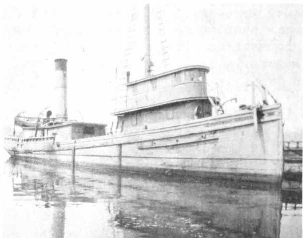
TREND IN POWERING OF MENHADEN BOATS IS EXEMPLIFIED IN THIS VETERAN VESSEL, WHICH WAS STEAM PROPELLED UNTIL 1938 AND THEN CHANGED TO DIESEL POWER
